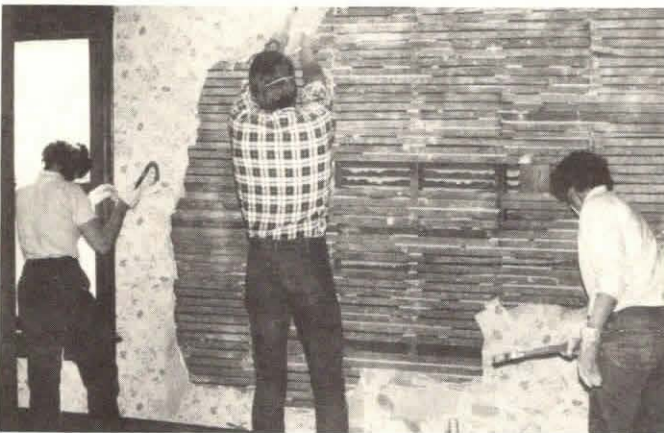
Historic Boulder volunteers demolish an interior wall of the organization's ROAR project house, Boulder, Colo. (J. Stowall)
