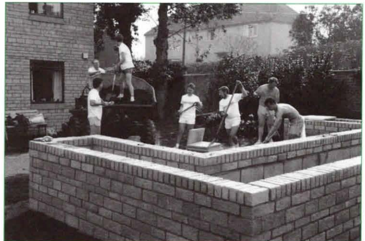
Volunteers from Allied Dunbar's Finance Division undertaking a 'Challenge' – building a raised garden at a residential home for elderly people.
