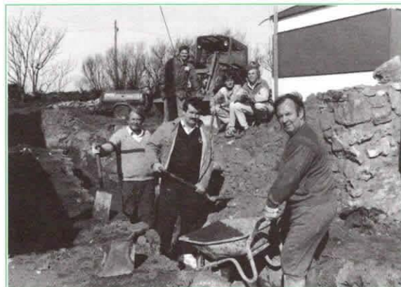
British Gas Wales – Men at hospice work
