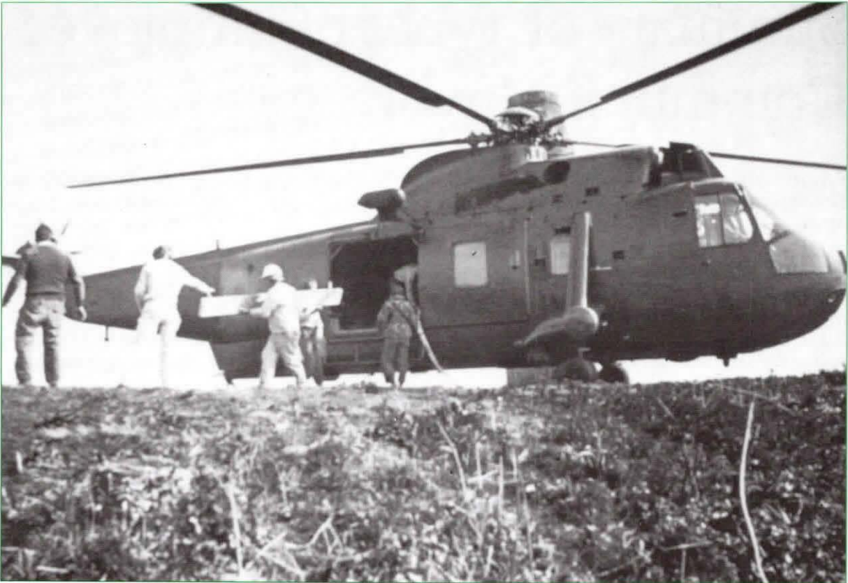
Royal Navy lifting stonemasons' equipment for restoration of a tower on St Michael's Hill, Montacute at the request of The National Trust
