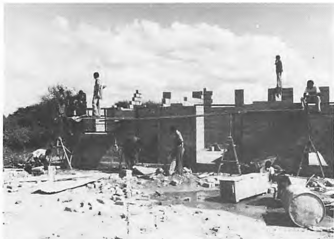
Members of the Tonota builders brigade construct their own warehouse.
