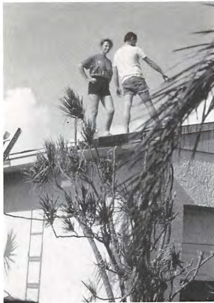
Doris Petersen, AAL district representative from Cutler Ridge, Fla., surveys damage to her roof with a volunteer.
