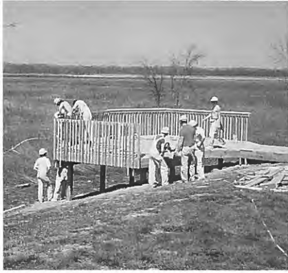
Building observation deck.
