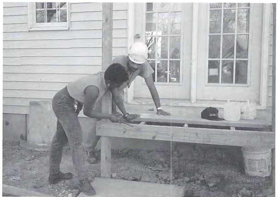
A HATT trainee learns to build a deck and do trimwork.
