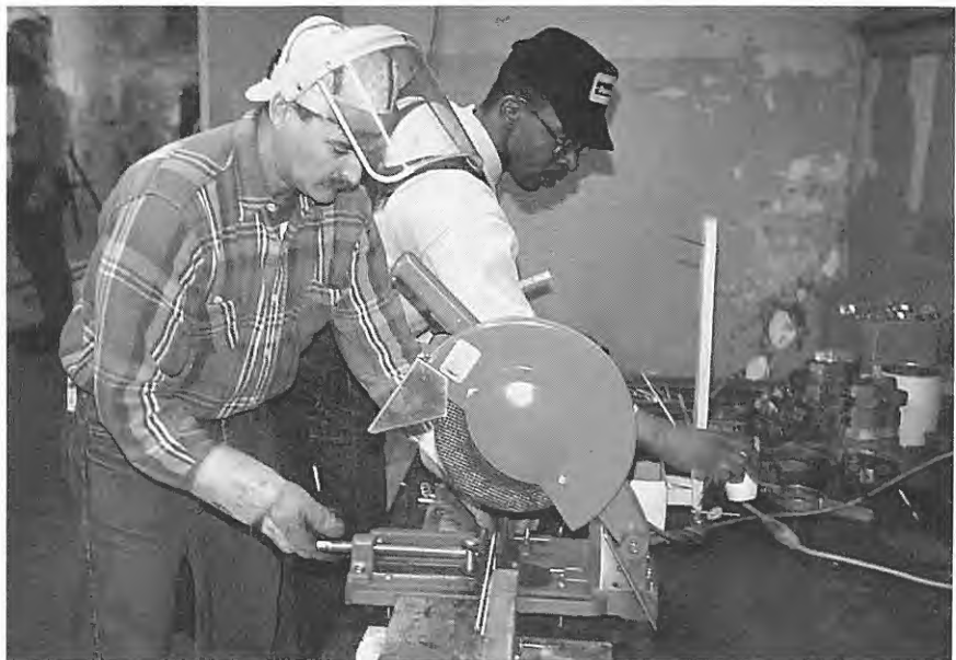
Union members at work on the Tom Geiger House for the homeless.
