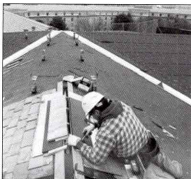
National Roofing Contractors Association, Sept. 11 winner
